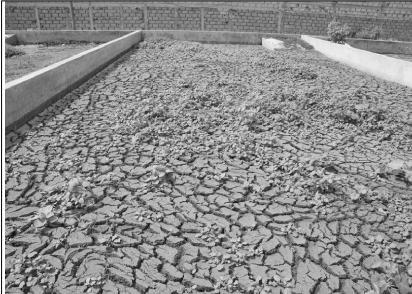
Figure 4 Faecal sludge drying bed currently in operation at Cambérène Faecal Sludge Treatment Plant in Dakar.
